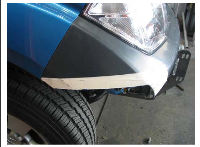
Figure 2: Use a jigsaw to cut the marked side of the bumper cover.
